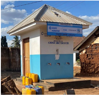
Prepaid water kiosks WOP Morogoro Urban Water Supply and Sanitation Authority
